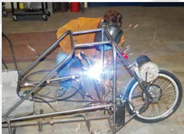
Top: MacKayla Koehn displays her design for this year's electric vehicle. Right: Karlee Logan welds the final pieces on the seat brace in this year's electric car.
